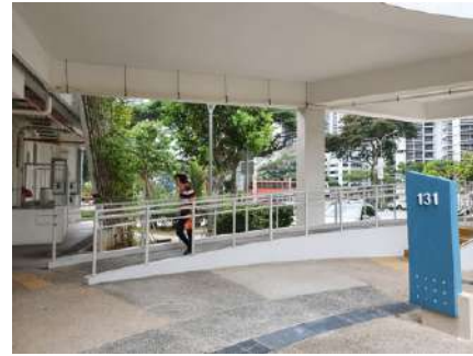
Figure 14: Close up of ramp
